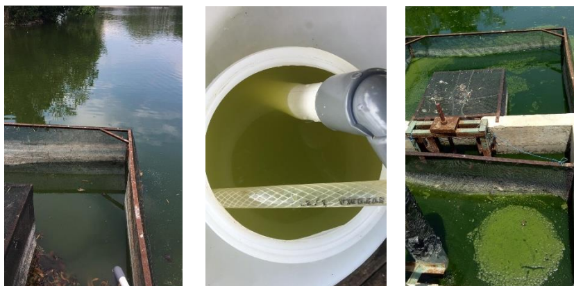
Gambar 2 Intake Pilot Plant ITDC Nusa Dua Area Lagoon
